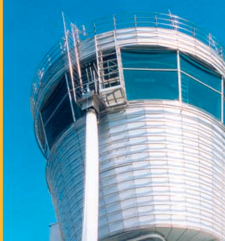
The Ingström Escape Chute hanging from the air traffic control tower at the Helsinki airport.
